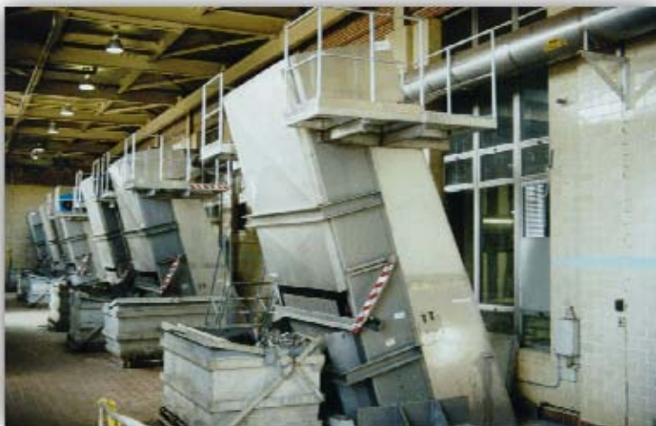
FC FRONT CLEANED MECHANICAL BAR SCREEN
